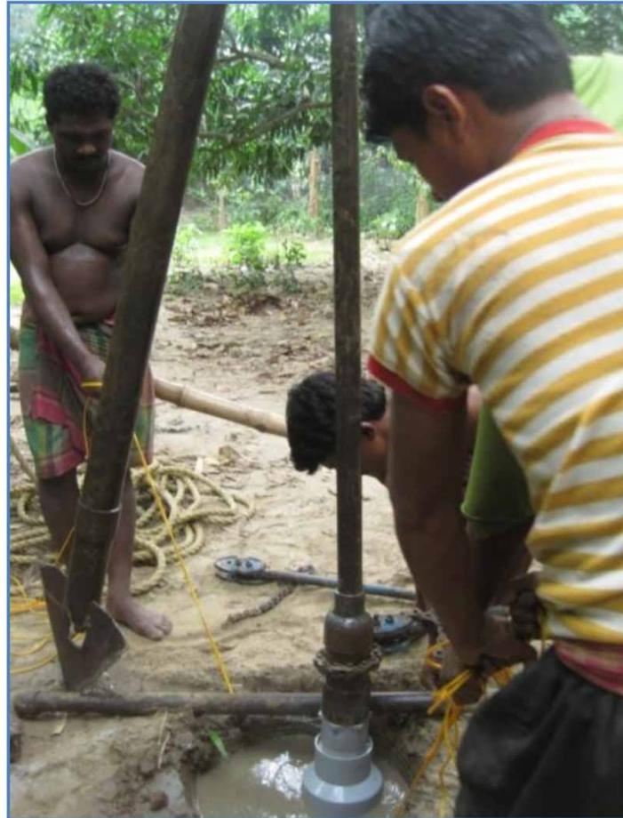
**Figure 3** | Lowering of the assembled 3 m by 25 cm PVC pipe into the 9 m by 46 cm hole.
